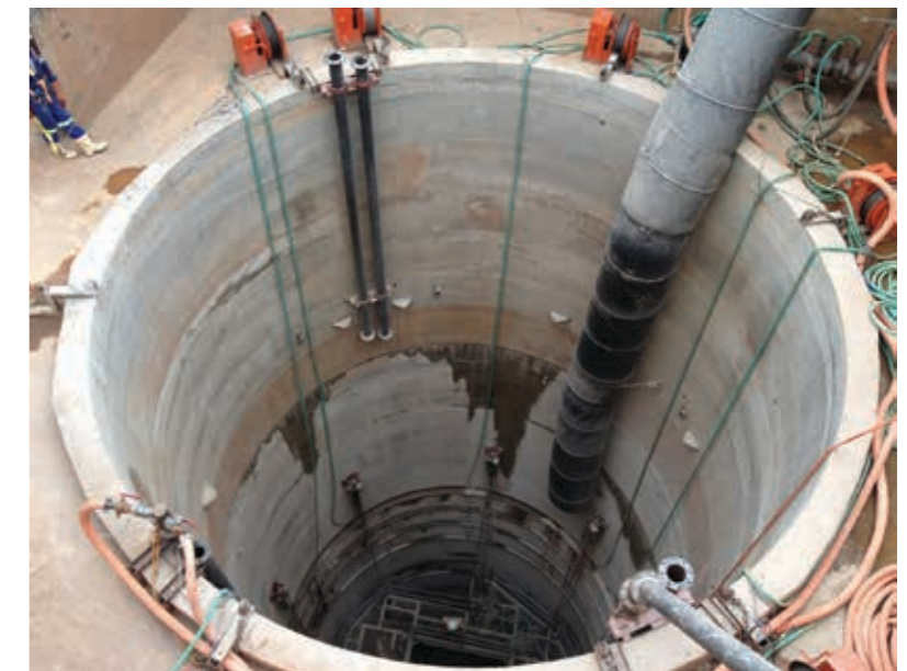
Sinking of a shaft barrel at a recent project in the DRC.
