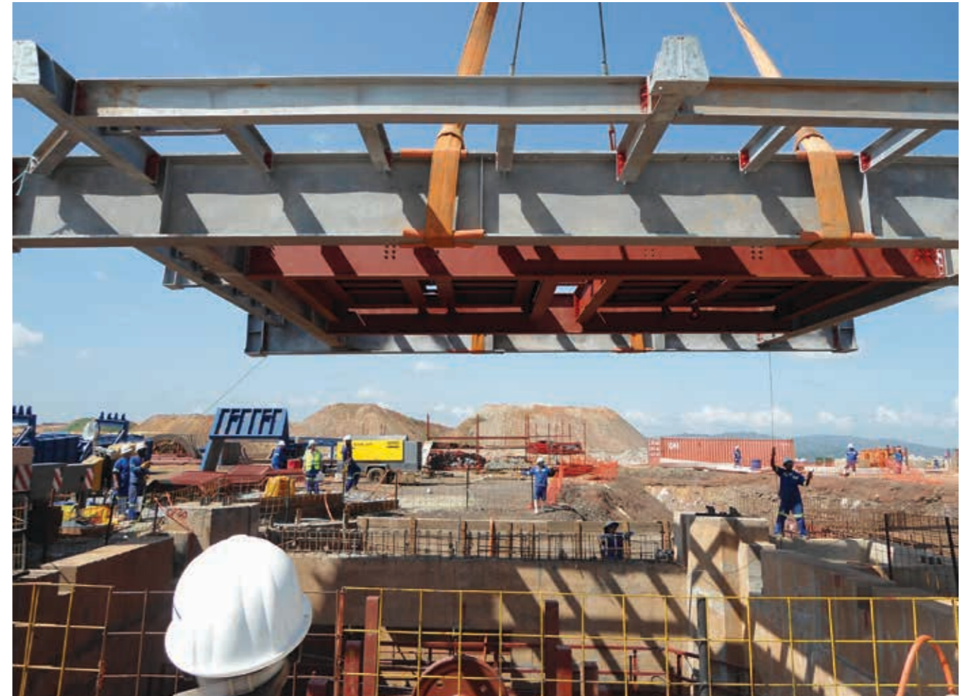
Head gear erection at a recent DRC project.
